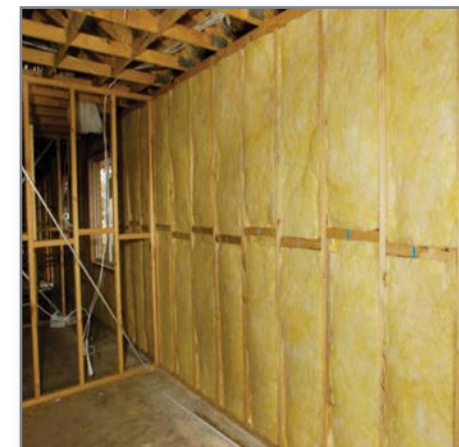
Insulation cut-outs for power points
