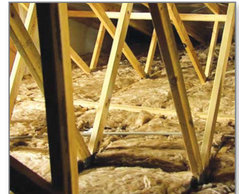
Fully installed ceiling insulation batts - no gaps
