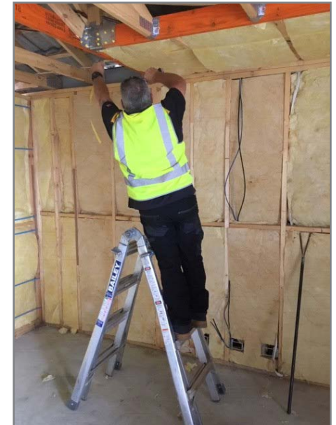
Example of fitting edge batts
