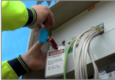
Fixing power sign to meter box
