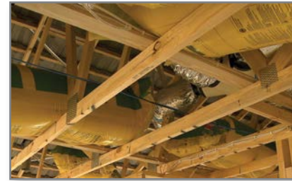
Preload packs and distribute in ceiling space
