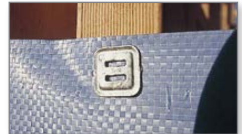
Wall wrap fixing fastener
