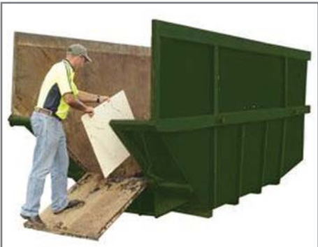
Removing off-cuts from site
