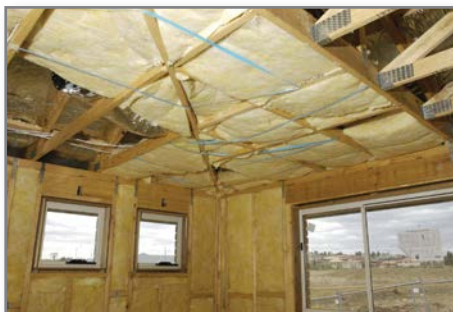
Example of ceiling insulation in progress using stringing
