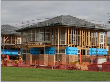
Safety rails fitted for working at heights
