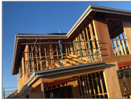
Roof edge fall protection.
