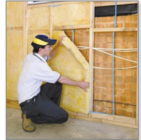
Examples of well installed wall batts
