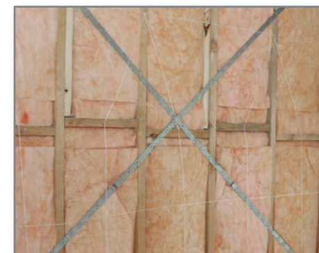
Using off-cuts to fill spaces above and below noggings
