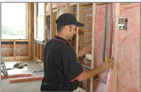
Installing insulation behind services
