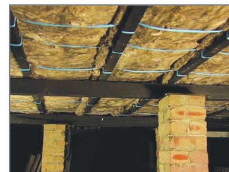
Stringing under floor insulation in place
