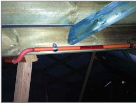
Exposed cables - not compliant
