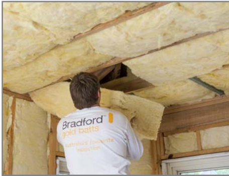
New build - Installing ceiling insulation prior to ceiling installation.
