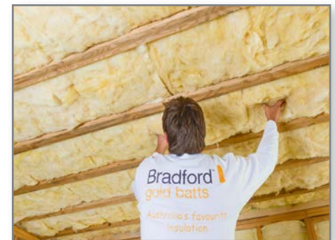
Installing ceiling batts from underneath before ceiling linings are fitted.
