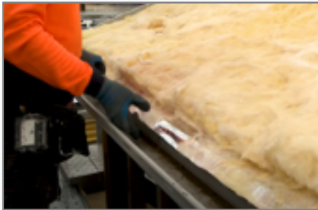
Trim back bulk insulation. Only overlap sarking into gutter
