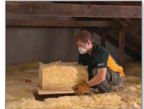
Check insulation installed over attic access cover
