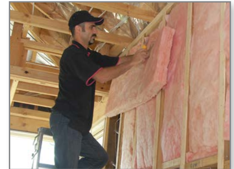
Examples of fitting wall batts
