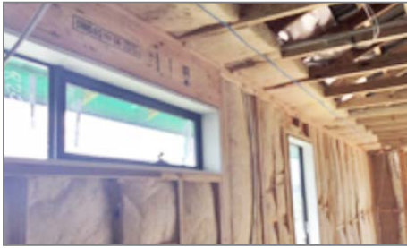
Installing perimeter batts over top plate
