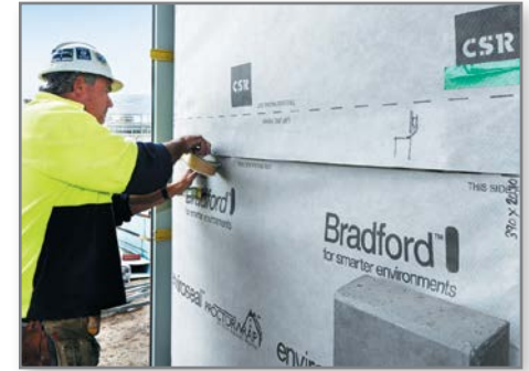
Taping and sealing membrane overlaps
