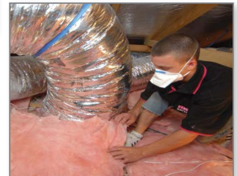
Fitting insulation snugly around ducting
