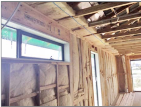
New build - perimeter batts installed.
