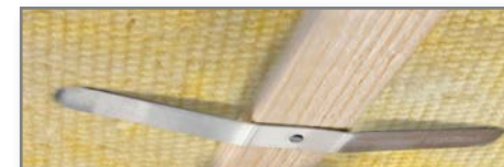
Butterfly clip holding insulation in place
