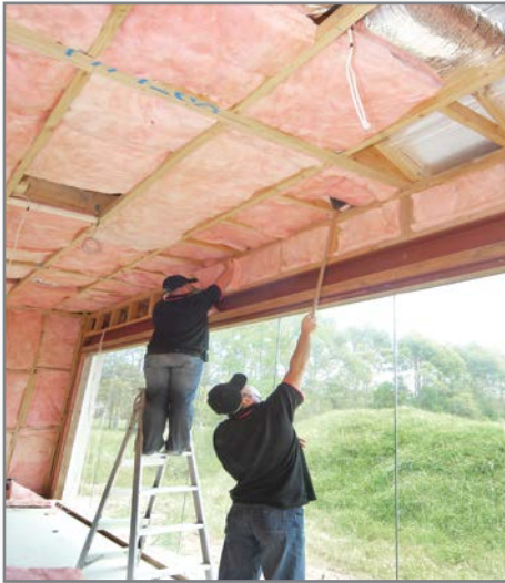
Installing insulation from underneath - note batts cut to fit above windows and over top plate
