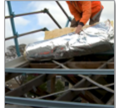
Vertical roll out over horizontal battens
