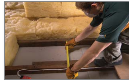
Measure - right sized batts
