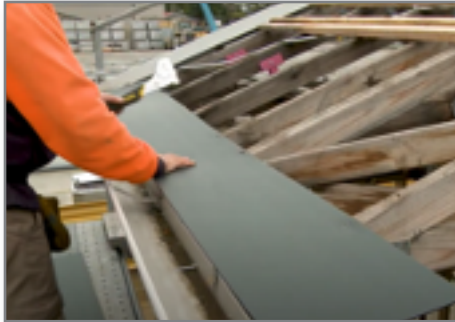
Fixing anti-ponding board
