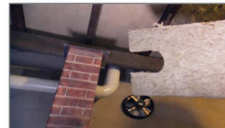
Cutting insulation around under floor services
