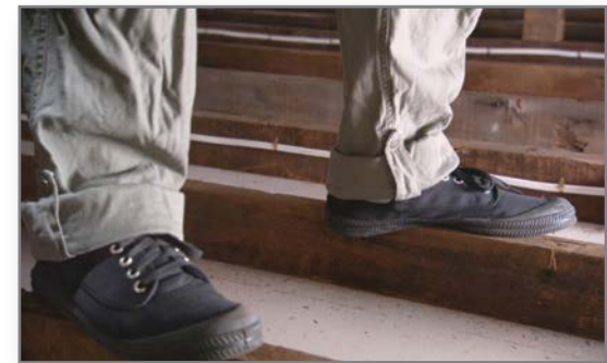
Using floor joists for safe footing
