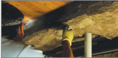
Cutting insulation to install around plumbing services
