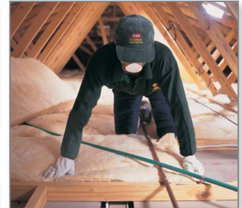
Install batts under services
