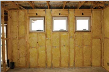
Installing insulation from underneath - note batts cut to fit above windows and over top plate
