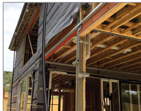
Elevated floor- installing insulation between floor joists
