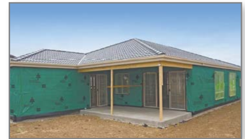
Wall wrap installed prior to windows being fitted
