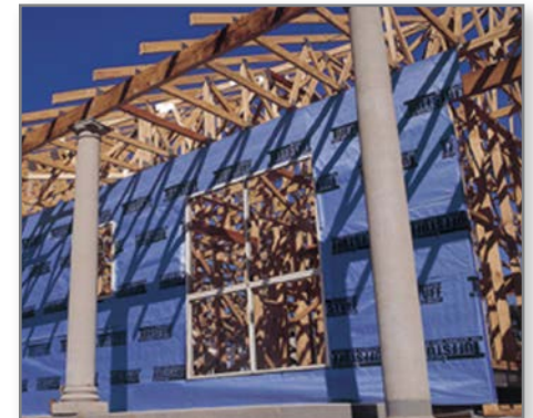
Fixing wall wrap neatly around windows
