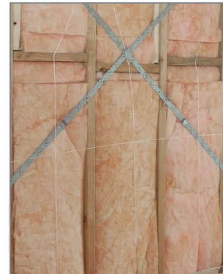
Bracing studs for internal walls and stringing in wall batts
