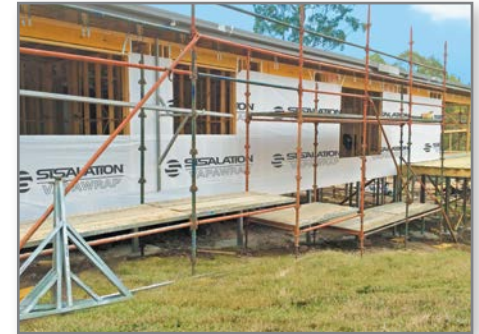
Wall wrap installed prior to windows being fitted
