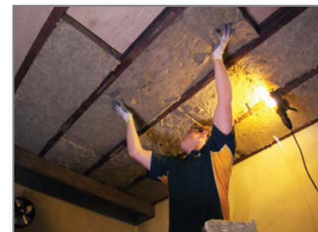
Elevated floor- installing insulation between floor joists
