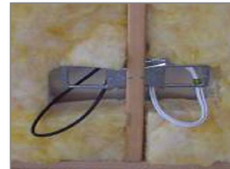
Insulation cut-outs for power points
