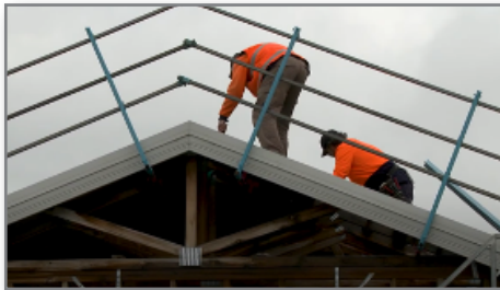
Start apply membrane from gutter line and work up to ridge
